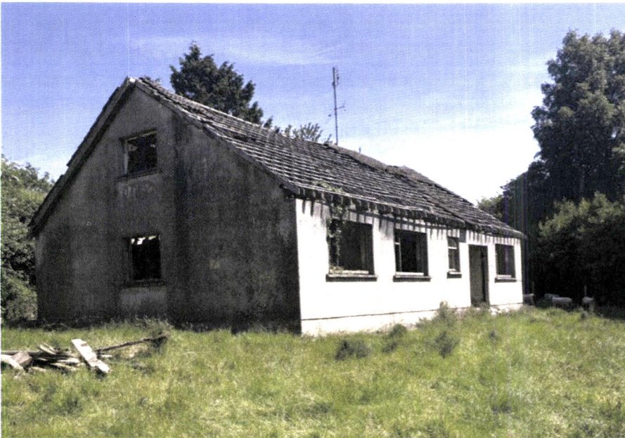
Fig. 4: Photograph of the existing dwelling structure with its windows and roof tiles removed for delayed maintenance (1)
